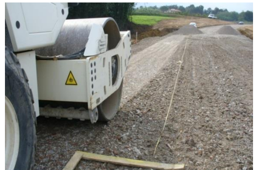
Fig. 3. Continuous Compaction Control of unbound C&D layers.
