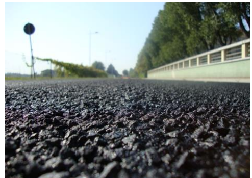
Fig. 1. Cold laid micro-surfacing.
