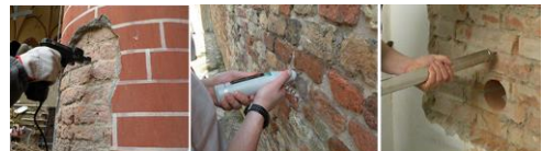
Fig. 4. On-site mechanical characterization of historic mortars by micro-destructive testing (Colla).
