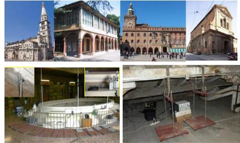
Fig. 1. Some structures recently surveyed: Ghirlandina tower and Modena Cathedral (UNESCO sites), Palazzina della Viola, Palazzo D'Accursio, San Barbaziano church (top); Palazzo Malvezzi, load tests on a ceiling, with details of traditional and wireless monitoring systems, and on a timber beam (bottom) (Colla).
